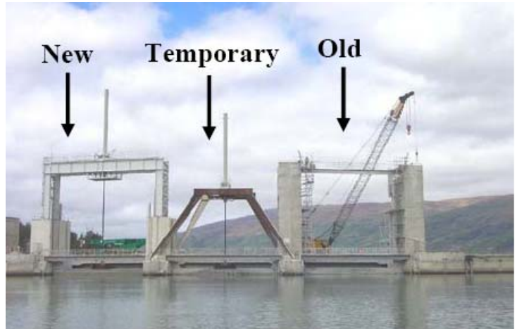
Figure 20. Roxburgh Dam spillway gantry upgrading
