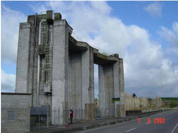
Figure 19. Whakamaru Dam strengthened spillway columns
