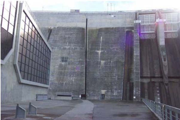
Figure 4b. Clyde Dam slip joint (courtesy Contact Energy)
