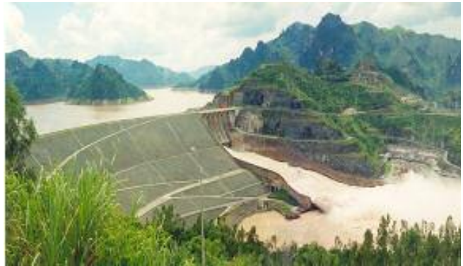
The HoaBinh Dam Le barrage de HoaBinh
