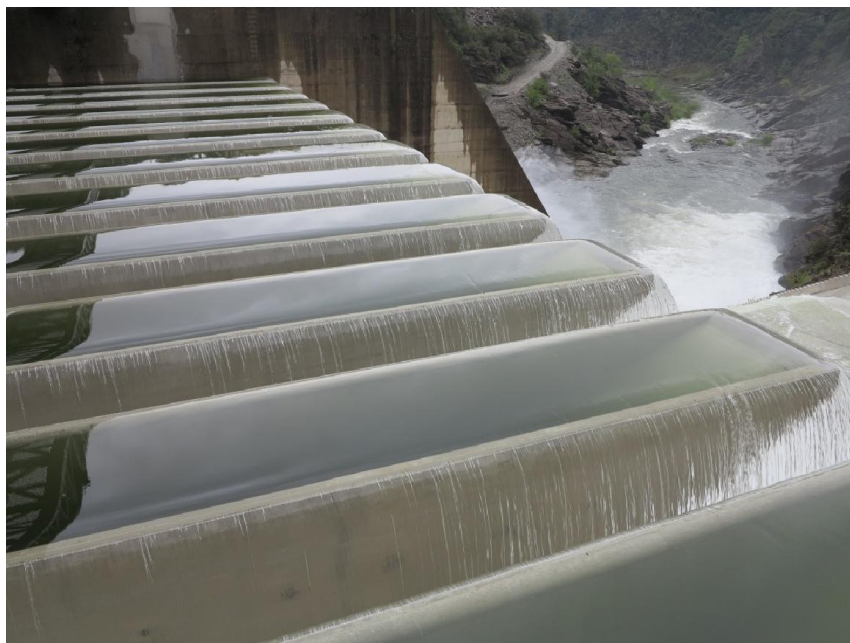
Figure 6.7 Flow over the Malarce dam PKW (France) with an upstream head of a few cm (Photo courtesy of EDF)
