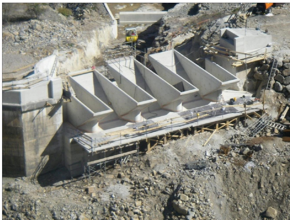
Figure 6.1 View of the PKW spillway of Gloriettes Dam in France during construction
