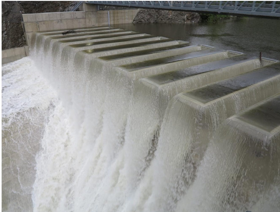
Figure 6.2 View of the PKW spillway of Malarce Dam in France during spillage
