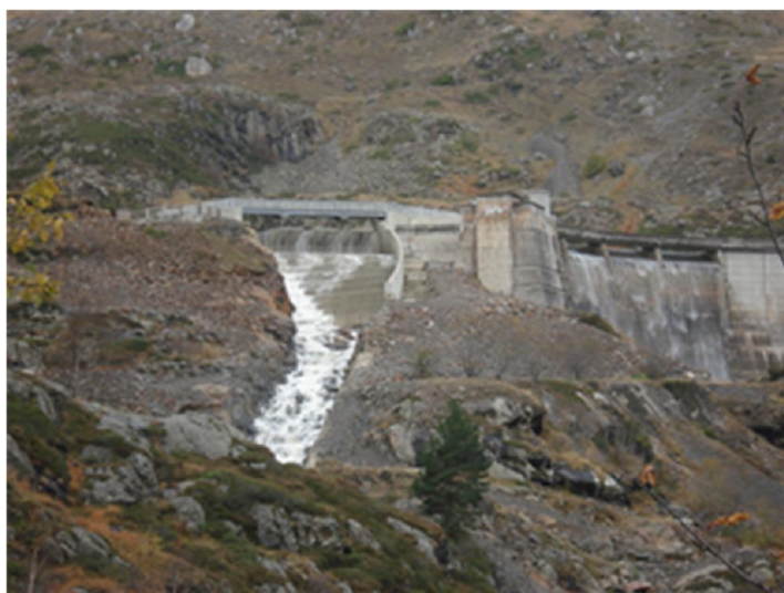
Figure 6.9 Low slope stepped spillway channel downstream of the Gloriette dam PKW (Photo courtesy of EDF)
