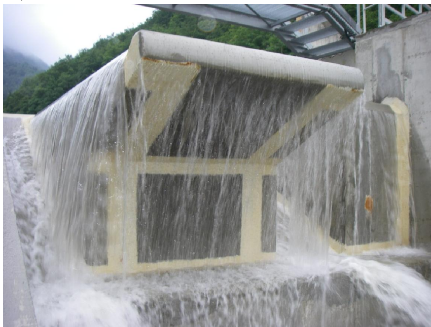
Figure 6.8 Flow over the Escouloubre PKW (France) with an upstream head of a few cm (Photo courtesy of ULg-HECE)
