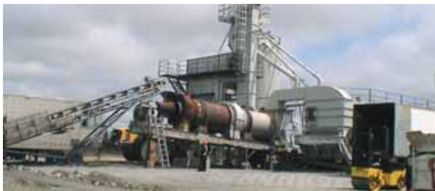
Construction of Nemiscau-1 Dam – The Asphalt Concrete (batch) plant
