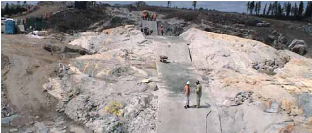
Nemiscau-1 Dam site – Rock excavation and concrete plinth
