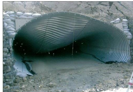
Fig. 3.8 Deformed culvert
