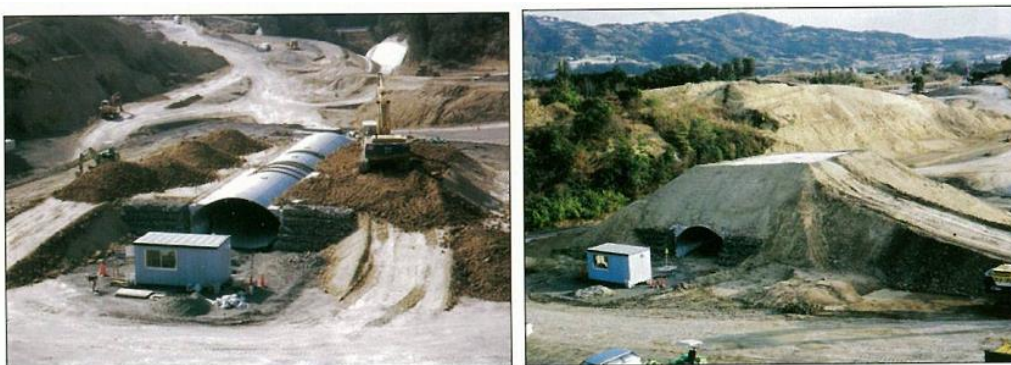
(c) Covering rock soil
