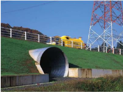
Fig. 1.1 Corrugated Drainage
