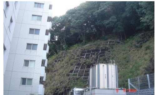
Fig. 12. Non-frame and concrete on Matsuyama Castle slope
