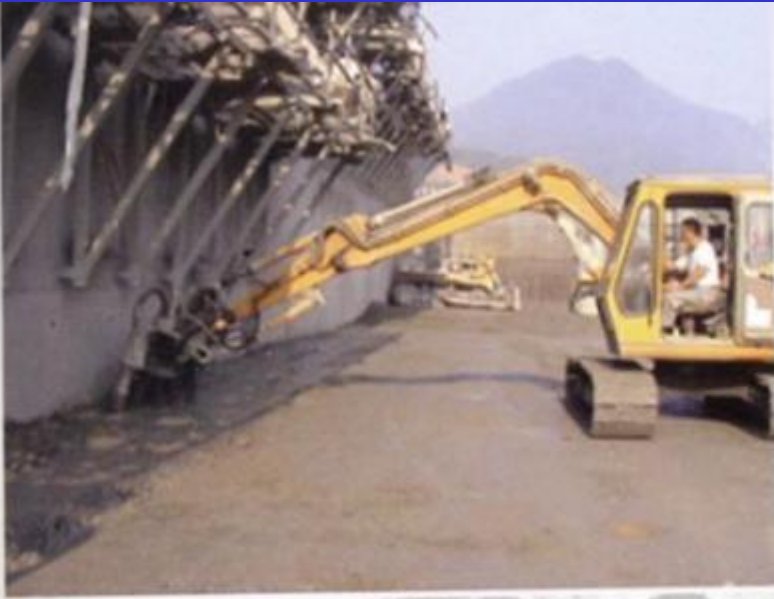
Vibrating of GEV RCC
