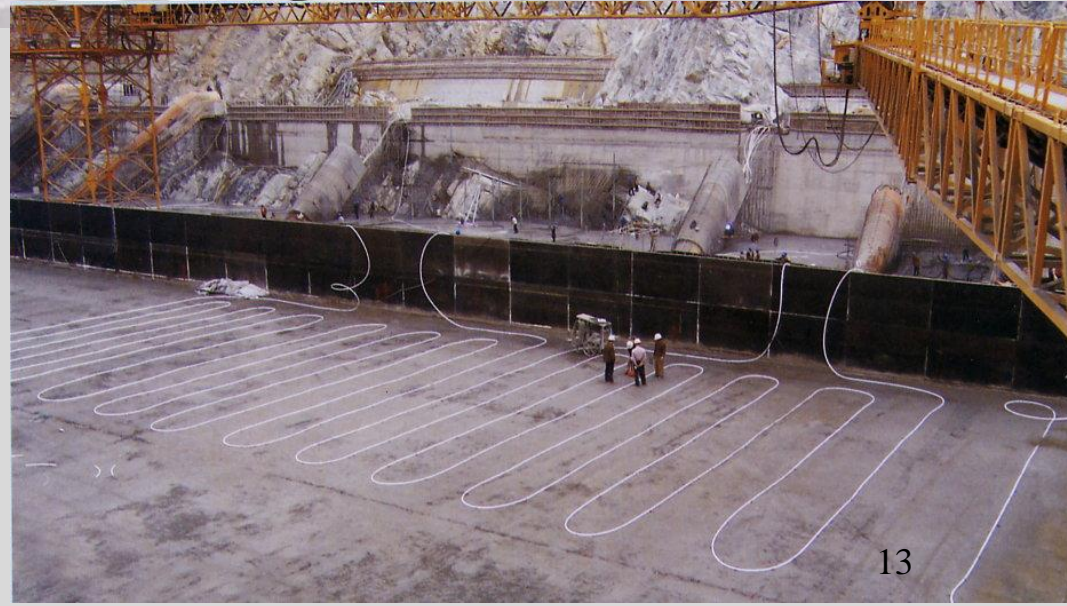
Internal cooling in large RCC dams
