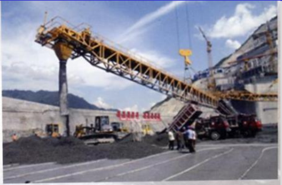
Pouring RCC with high speed belt feeding line
